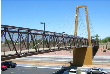
Loop 101/63rd Ave. Pedestrian-Bike Bridge
