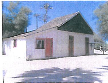
Adobe Building Sahuaro Ranch
